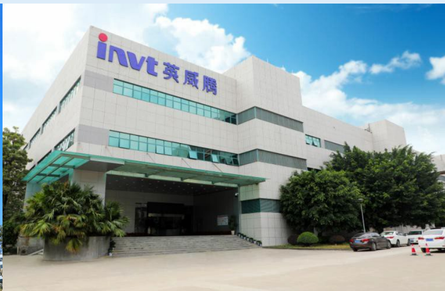
Shenzhen Fuyong Industrial Park
